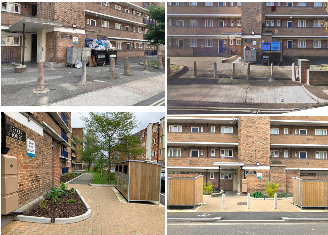
Some of the Elmington Estate de-paving and landscape improvements (Housing and Flood management joint scheme, through the Great Estates Program)
